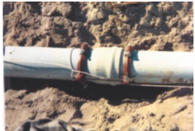
8" Series PVP restrainer installed by Kenborough Contracting on AWWA C-900 DR 18 PVC pipe in the Town of Markham, Ontario, Canada.
