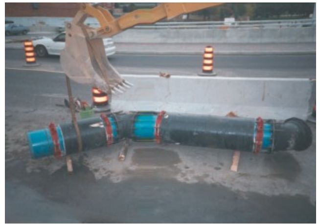
16" Series PVM restrainers completing 45° vertical offset above ground for bridge crossing at Regional Municipality of Sudbury, Ontario, Canada
